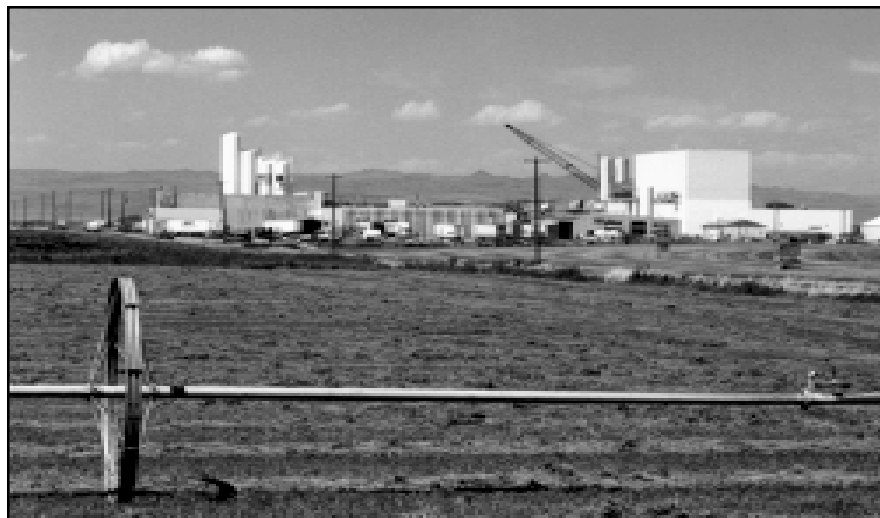
Cheese companies are following milk west, and most Western cheese companies are adding capacity to their current locations—as Avonmore is doing at this processing plant in Gooding, Idaho—or building new plants.
